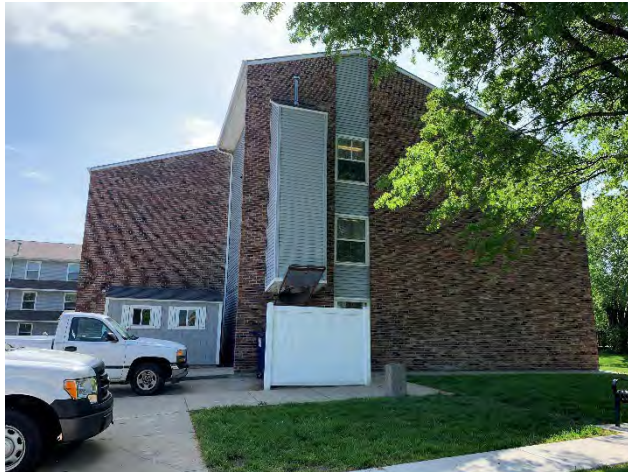
Looking east toward the building
