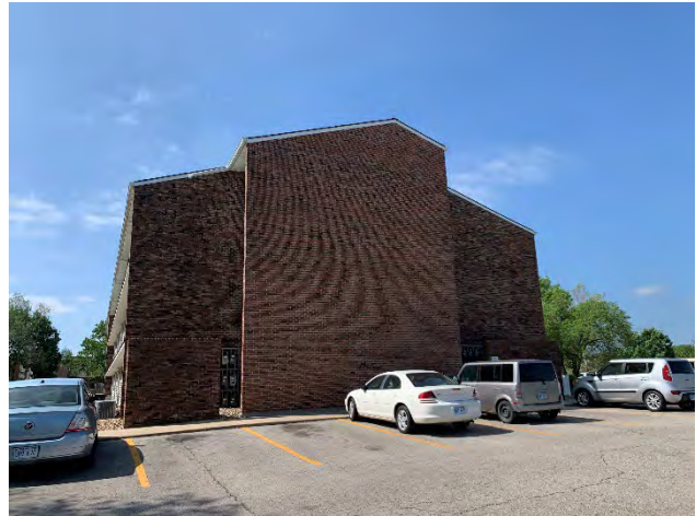
View looking south at the side of the building
