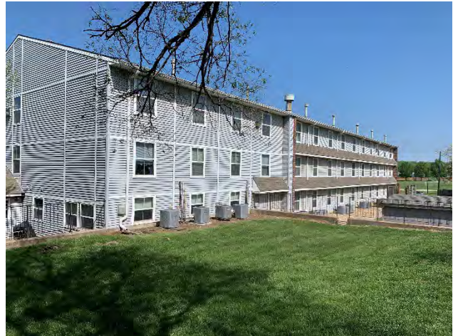
Looking northwest at the site
