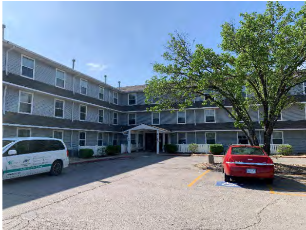
View looking south at the front of the building
